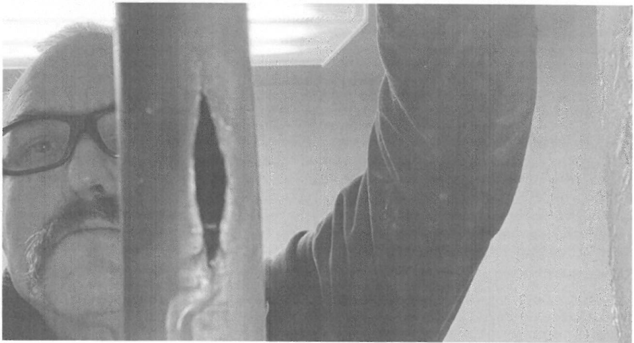
Figure 5. Water Pipe Break in the East Wall of Station 94
