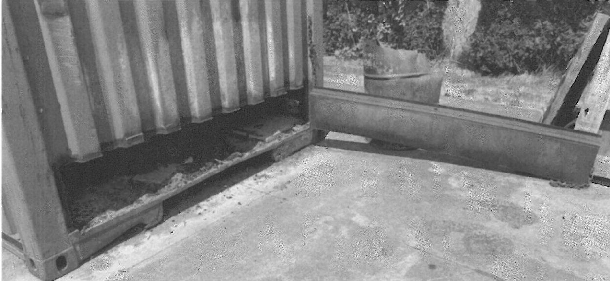
Figure 3. Cleanout Damage
